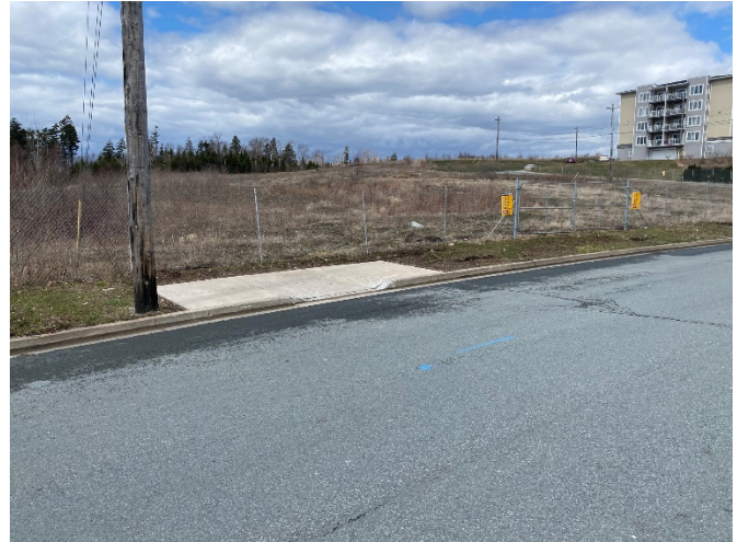
Photo 11-3: Concrete Pad at Location with Curb but No Sidewalk (Middle Sackville)
