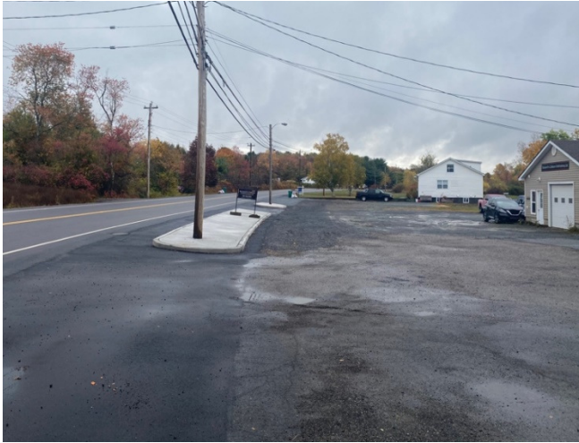
Photo 11-2: Concrete Pad Between Parking Lot and Road (Newport Corner)
