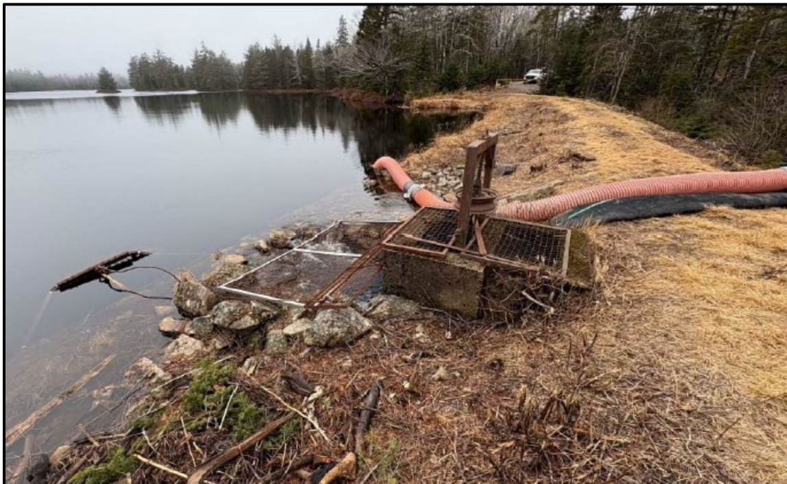
Figure 1-2. Existing Control Structure
