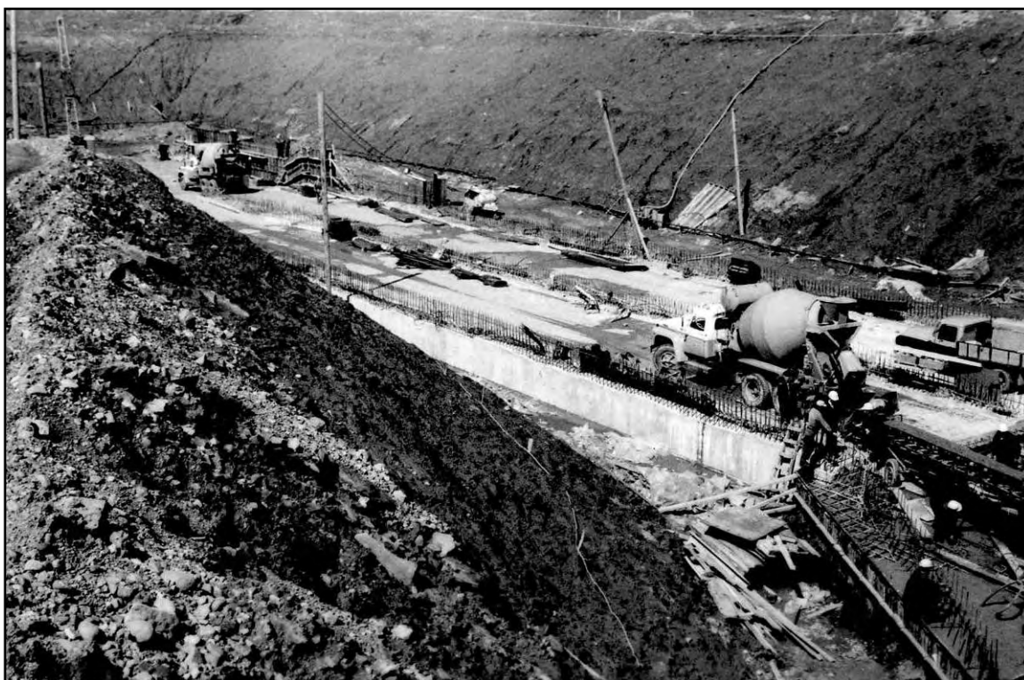
Figure 2.18: Construction of the floor of the new tide gate channel in late 1969 (photo from MMRA Archives 1969).
