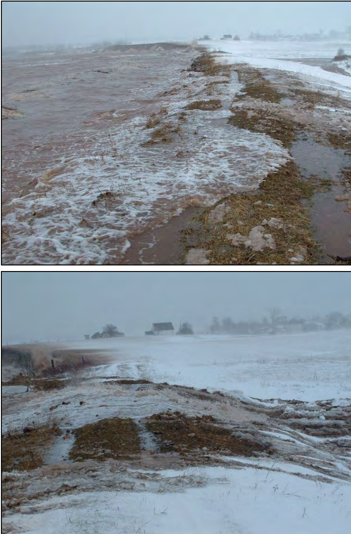
Figure 2.6: Storm impacts on Feb 1, 2006 at the Avonport Dyke. a) storm waves battering marsh; b) storm surge reached upper limits of dyke and dyke overtopped. Photo by T. Hamilton, 2006.
