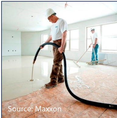
Figure 7: Gypsum Self-Leveling Floor
