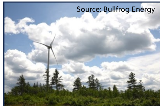
Figure 4: Ellershouse Wind Turbine
