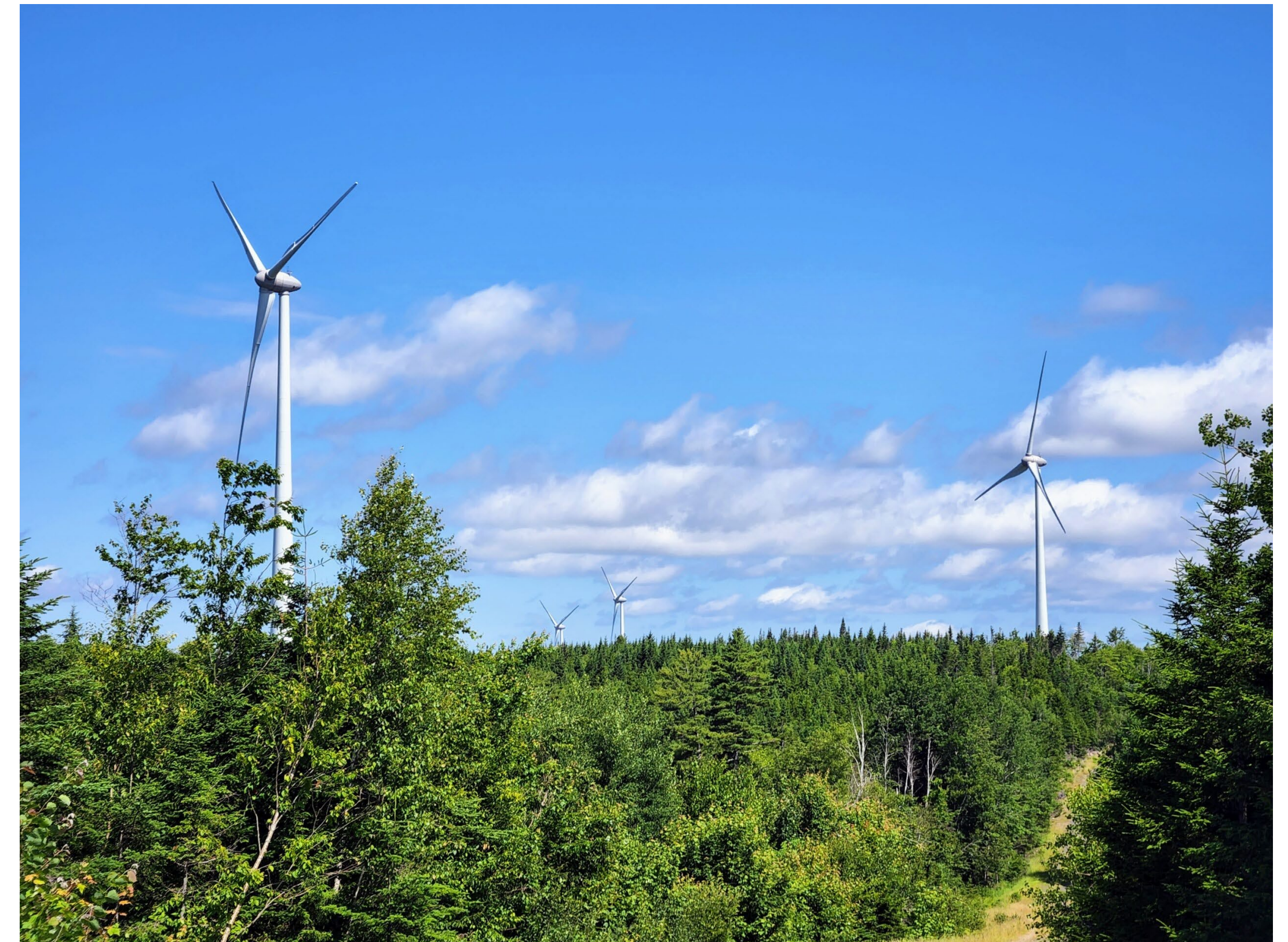
Ellershouse I & II Wind Farm, photo is property of AREA
